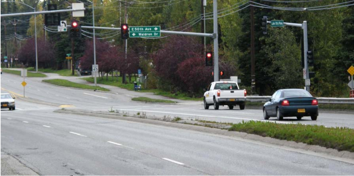
Waldron and E.50 th intersections from the SW. The left turn pocket with the light forms a continuous divider with the dividers at 53 rd .
