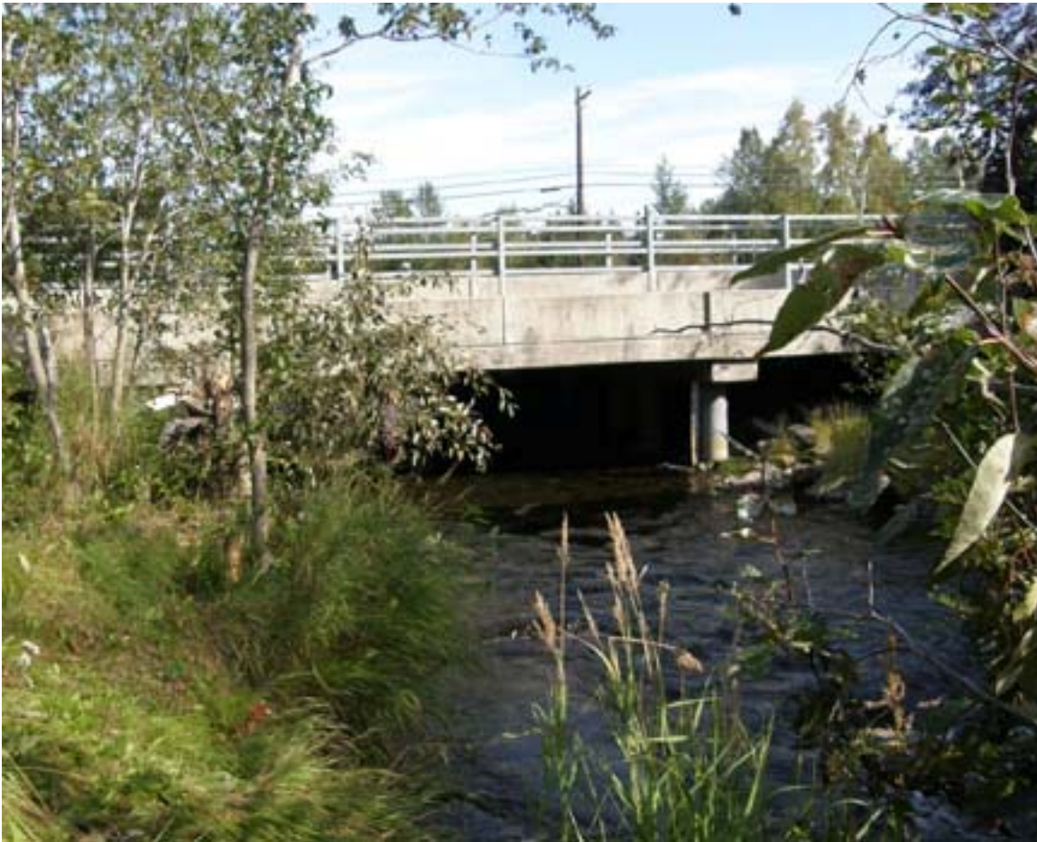
Car bridge over Campbell Creek from the west.
